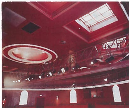
Another view showing curved and main lighting bridges.
