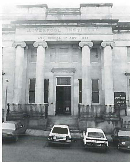
LIPA's imposing entrance is a gateway from the past that leads to a technological future.
